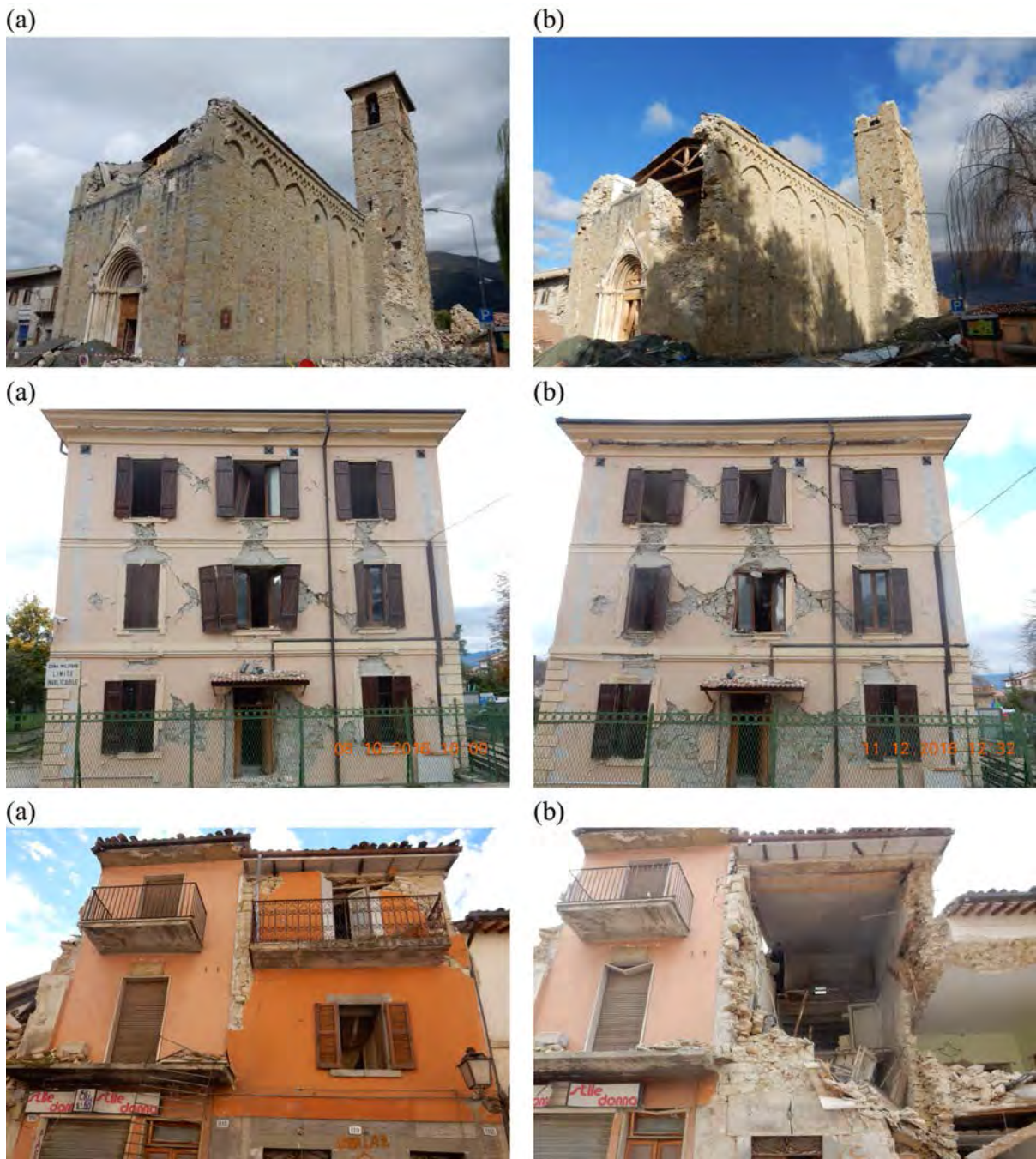
Figure 17. Incremental structural damage of the church of Sant’Agostino (top), the local police station (middle) and one of the several masonry buildings collapsed after (a) the event of 24 August earthquake and (b) the entire sequence.
