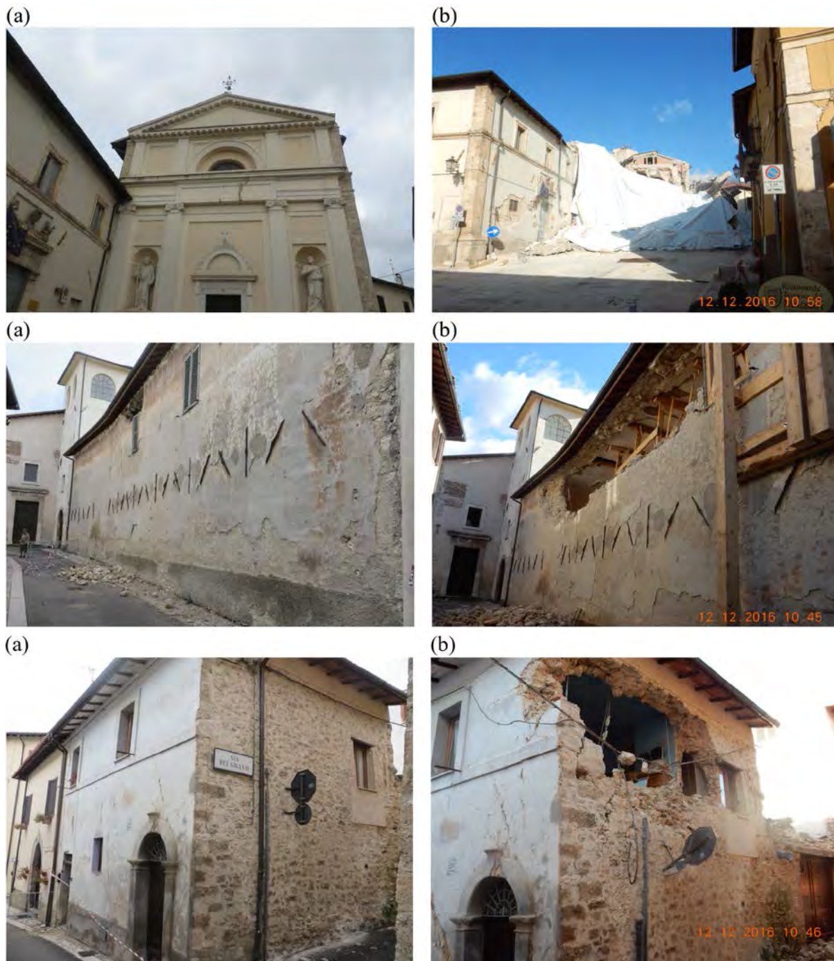
Figure 20. Seismic damage observed in characteristic masonry buildings (a) after the 24 August earthquake and (b) at the end of the entire seismic sequence.
