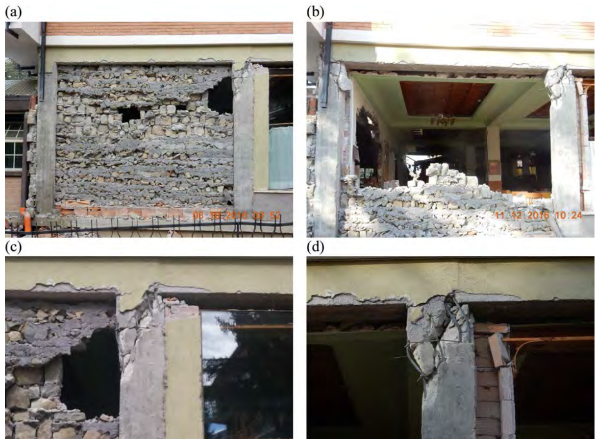
Figure 13. Reinforced concrete residential building (a,c) after the 24 August earthquake and (b,d) after the entire sequence. (a,b) External infill failure and (c,d) shear failure at the column top.
