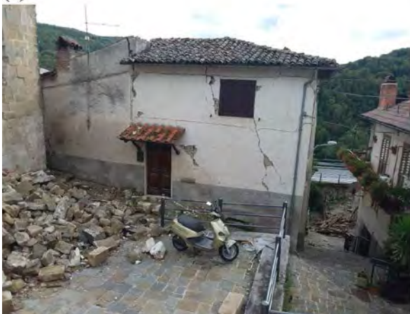
Figure 10. Masonry residential building: (a) after the first earthquake; and (b) after the sequence.
