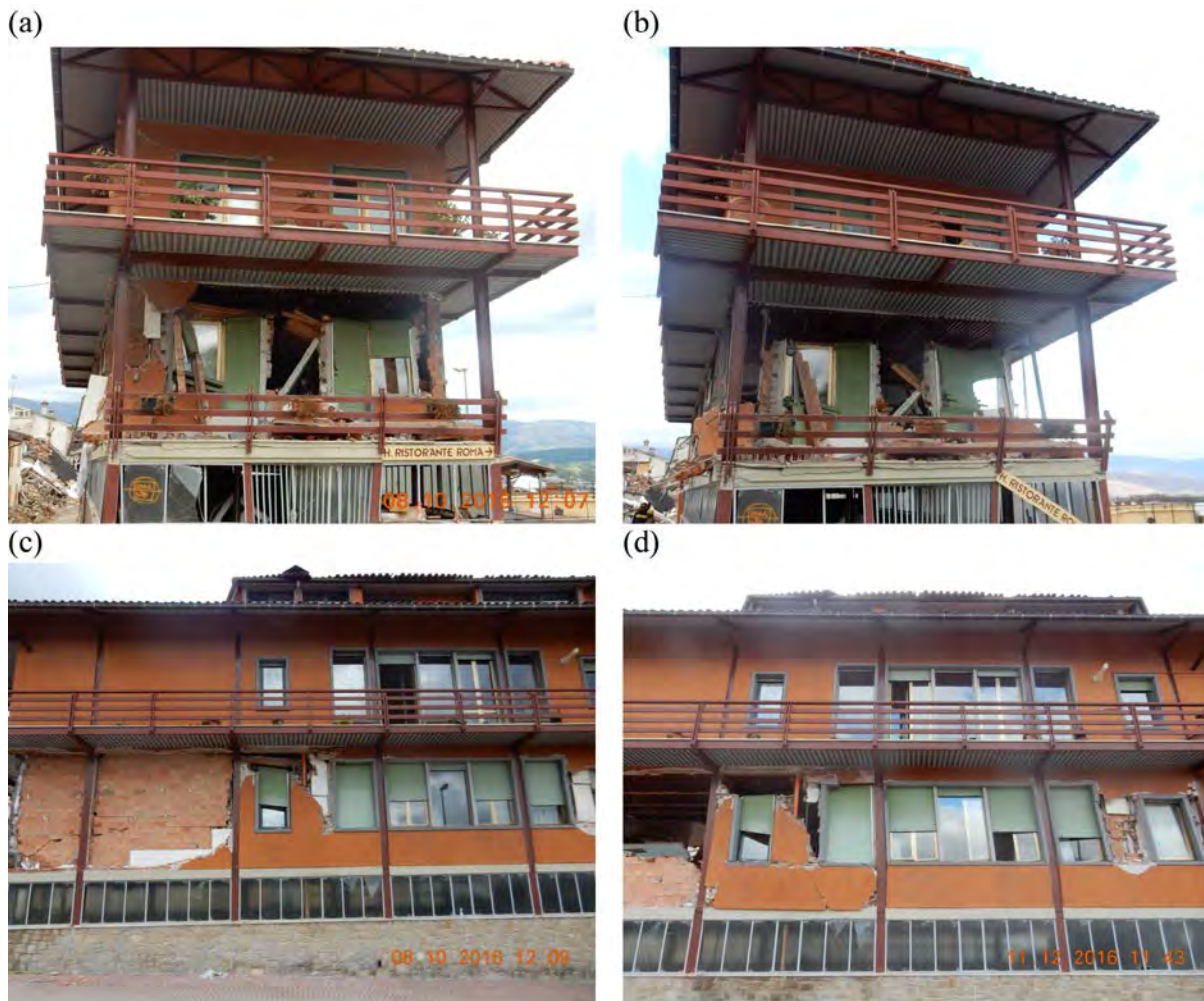
Figure 16. Steel residential building. (a,c) Limited damage after the 24 August earthquake and (b,d) extensive damage of the infill panels at ground level with evident residual drift after the entire sequence.
