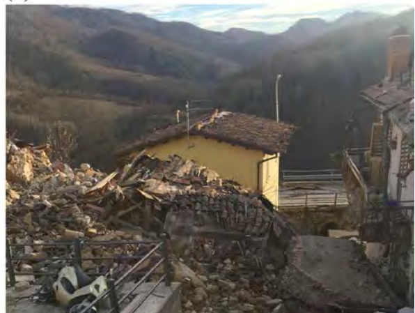
Figure 10. Masonry residential building: (a) after the first earthquake; and (b) after the sequence.
