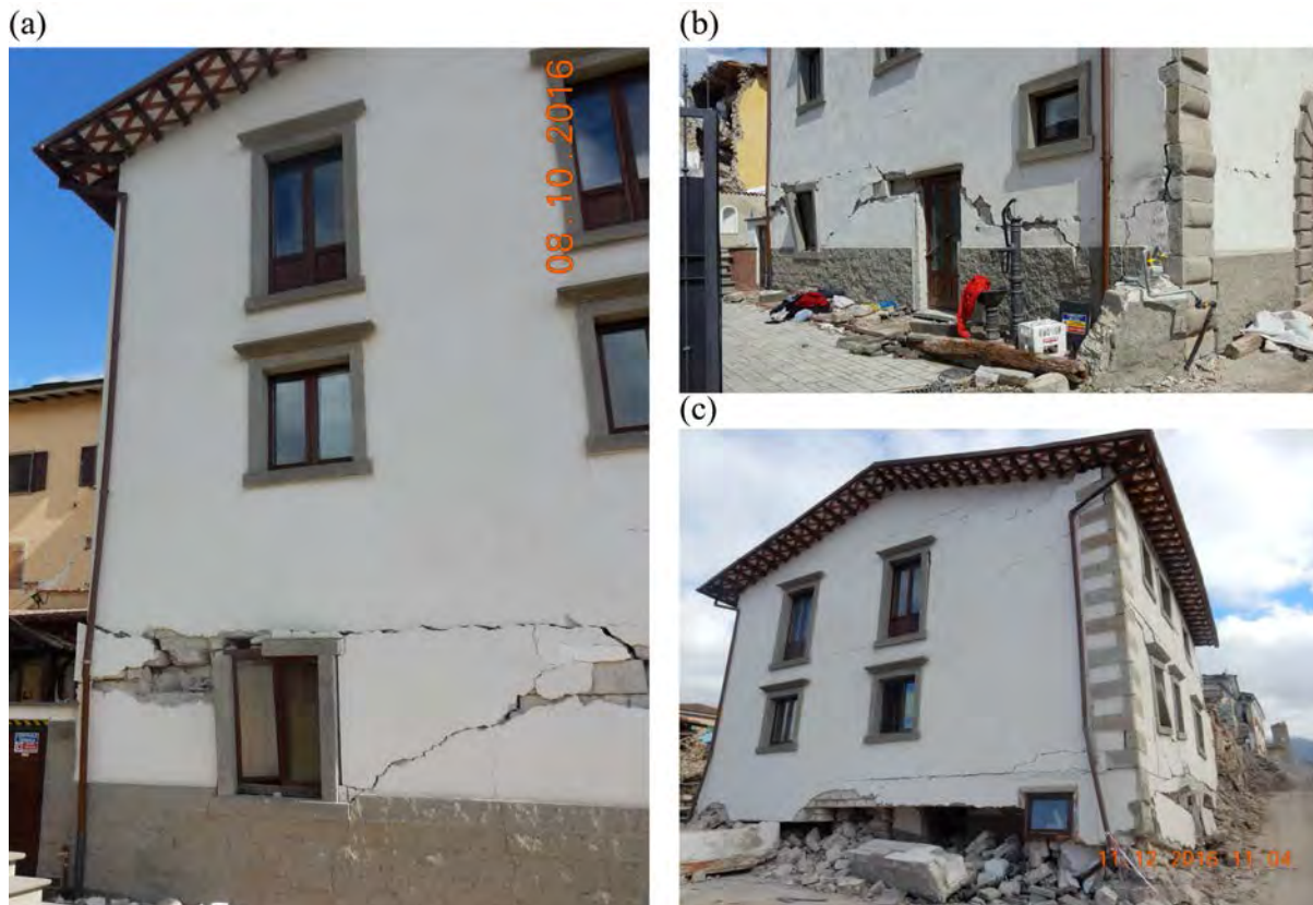
Figure 18. Residential masonry residential building after the 24 August earthquake (a, b) and (c) after the entire sequence. Shear failure of the ground floor bearing wall leads to soft story collapse at the end of the third event.
