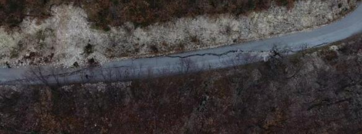
Figure 14: Aerial photograph of the Valle di Panico landslide (from GEER, 2017).
