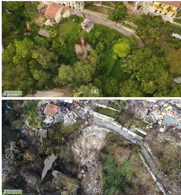
Figure 32: 3D model of the failure observed in area #5 in Figure 28 following: (a) the 24 August and (b) the 30 October event (from GEER, 2017).
