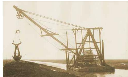
Clamshell Dredge Building a Levee – [SFEI, 2012]
